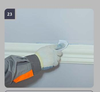
Wipe the excess adhesive with a cloth wetted with water if using «Evroplast Mounting» adhesive; with acetone if using «Evroplast Multipurpose» adhesive.
