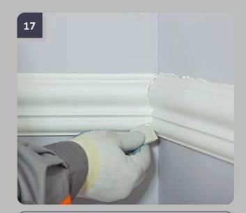
Immediately after attaching, remove excess adhesive using putty knife.
