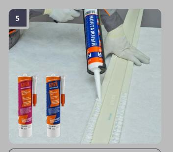
Apply «Evroplast Mounting» adhesive on the mounting surface or «Evroplast Multipurpose» adhesive along the length of the product. The thickness of the applied layer of adhesive shall be 3-5 mm.
