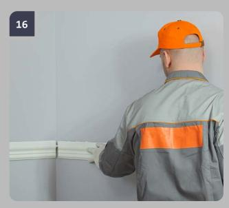
Press the product to the wall so that adhesive exudes from under the whole surface of junction. While moving the product along the wall, push it to the adjacent product so that adhesive exudes from the joint.
