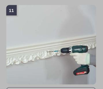
For products of more than 100 mm height, additional fixation with self-tapping screws at a spacing of about 600 mm is required.
