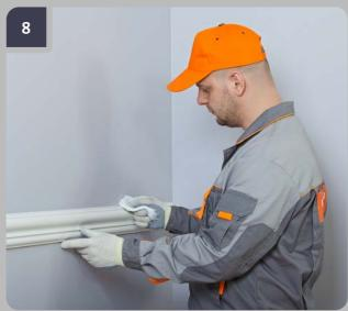
If necessary wipe the area of junction between the product and the wall with a cloth wetted with water if using «Evroplast Mounting» adhesive; with acetone if using «Evroplast Multipurpose» adhesive.
