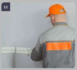
Cut the next product. Check the joining of the pattern and the profile of products, if necessary redo the cut.
