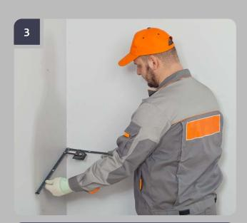
Using angle finder measure the angle of the corner of the room.
