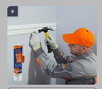
If using «Evroplast Mounting» adhesive it is necessary to hold it with finishing nails hammered under the product to prevent the product from sliding. The nails are removed after 24 hours.
