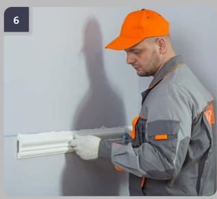
Affix the product to the place of installation according to the marking on the wall. Press the product along the whole length so that adhesive exudes from under the whole junction surface.
