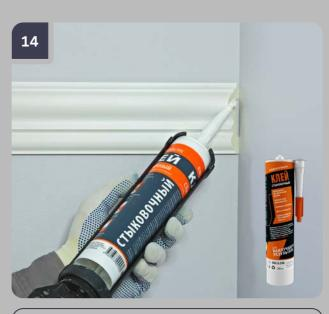
Apply «Evroplast for bonding joints» adhesive on the end surface of already mounted product.
