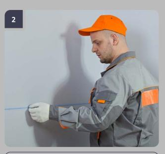
Using chalkline connect the marks along the perimeter of the room.
