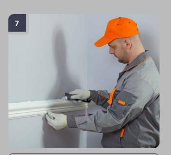
Immediately after attaching remove excess adhesive using putty knife.
