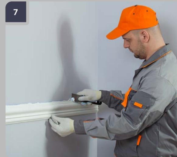
7 Immediately after attaching remove excess adhesive using putty knife.
