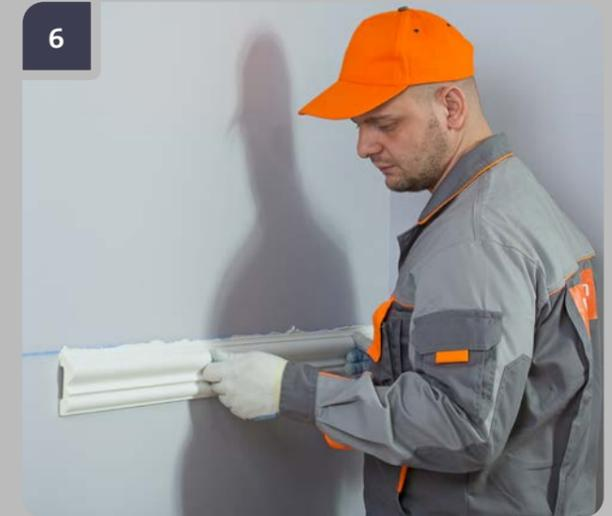
6 Affix the product to the place of installation according to the marking on the wall. Press the product along the whole length so that adhesive exudes from under the whole junction surface.
