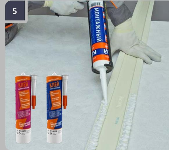
5 Apply «Evroplast Mounting» adhesive on the mounting surface or «Evroplast Multipurpose» adhesive along the length of the product. The thickness of the applied layer of adhesive shall be 3-5 mm.
