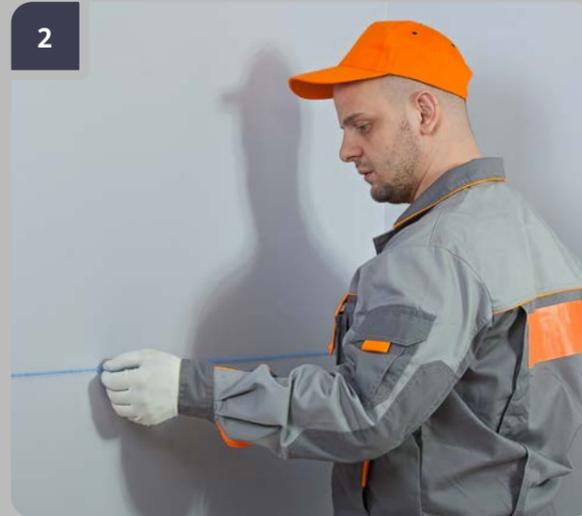
2 Using chalkline connect the marks along the perimeter of the room.
