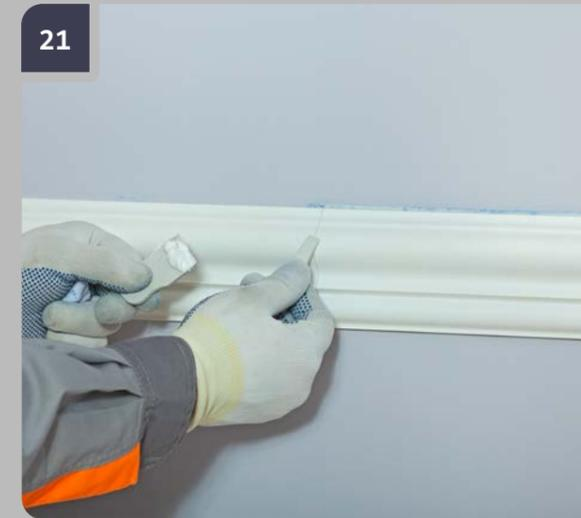
21 Fill the sanded joints with fine-grained, water-soluble filler for interior works, if necessary repeat "Step 20" until you get a flat surface.
