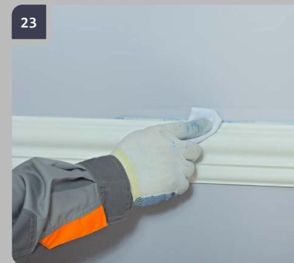
23 Wipe the excess adhesive with a cloth wetted with water if using «Evroplast Mounting» adhesive; with acetone if using «Evroplast Multipurpose» adhesive.
