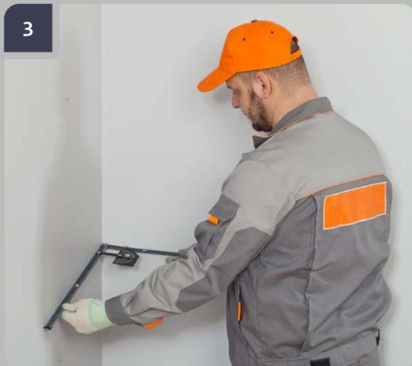
3 Using angle finder measure the angle of the corner of the room.
