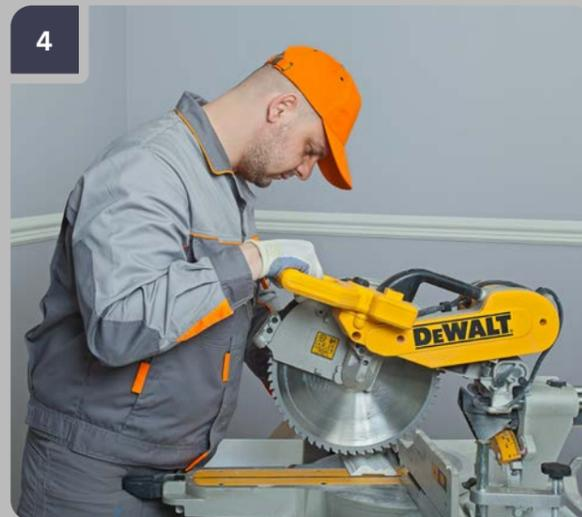
4 Set the angle on the trimming saw, make a cut on the product. In rooms with 90° corners it is possible to use a mitre box and a hand saw.
