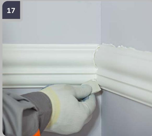
17 Immediately after attaching, remove excess adhesive using putty knife.
