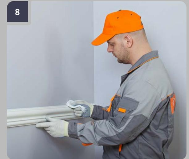
8 If necessary wipe the area of junction between the product and the wall with a cloth wetted with water if using «Evroplast Mounting» adhesive; with acetone if using «Evroplast Multipurpose» adhesive.
