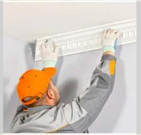
Remove emerged excess adhesive. Complete binding occurs upon expiry of 24 hours
