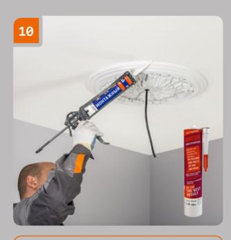
Fill the spaces in the junction area between the cornice and the walls/ ceiling, where the adhesive has not shown on a surface.
