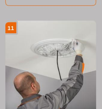
Wipe the area of the junction with a wet cloth. Wet the cloth with water if Assembly Adhesive is used and with Acetone in case of using Multipurpose Adhesive or Adhesive for bonding joints.
