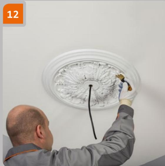
Paint following the instruction of paint producer the rose and ceiling in case of need.
