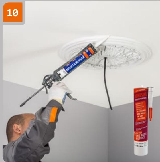
Fill the spaces in the junction area between the cornice and the walls/ ceiling, where the adhesive has not shown on a surface.
