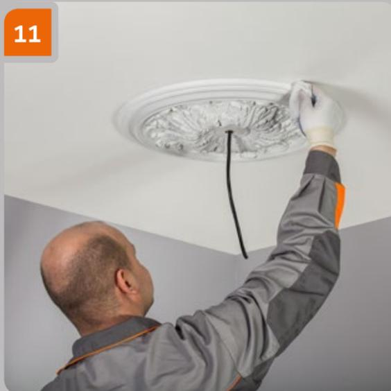
Wipe the area of the junction with a wet cloth. Wet the cloth with water if Assembly Adhesive is used and with Acetone in case of using Multipurpose Adhesive or Adhesive for bonding joints.
